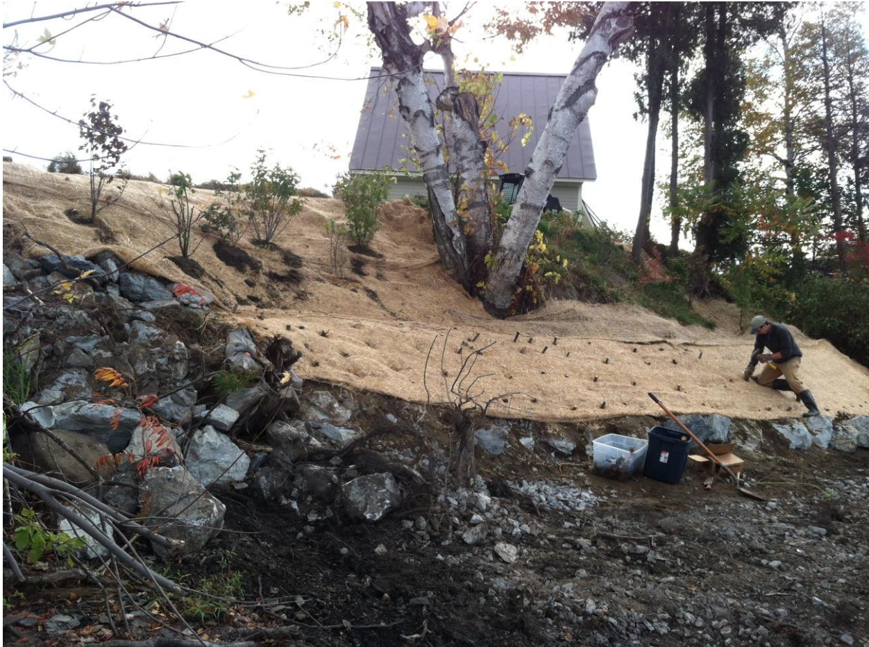
Figure 16. This shoreland restoration project occurred after catastrophic flooding on Lake Champlain in 2011. By re-vegetating the shore with native live tree stakes and fiber mats, the bank is better stabilized than the neighboring shoreland area that utilized solely stone riprap. Photo credit: Northwest Regional Planning Commission
