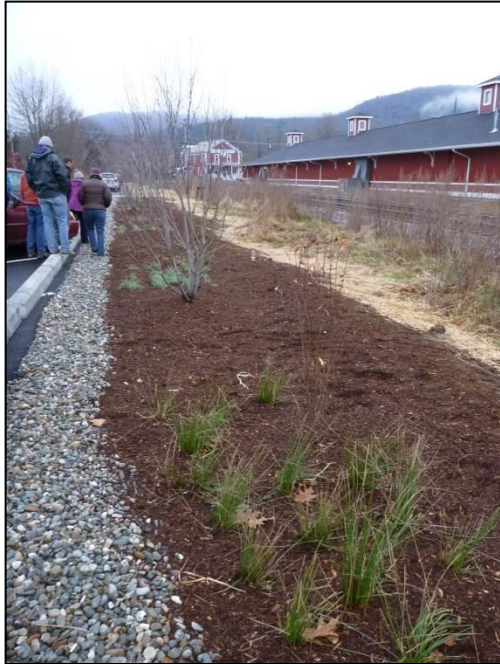
Richmond parking lot bioretention area.
