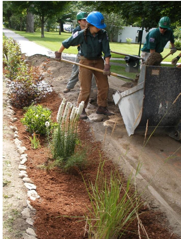
Figure 6. The Vermont Youth Conservation Corps (VYCC) installed this Rain Garden in St. Albans City with ERP funding. Photo credit: VYCC
