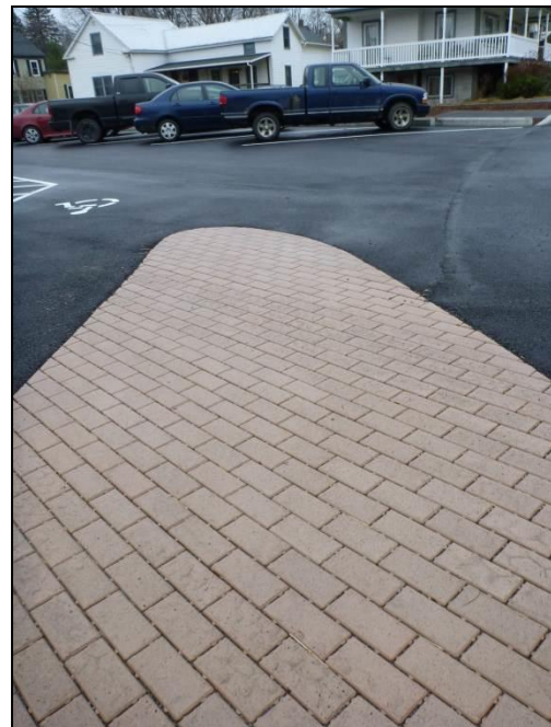
Richmond parking lot permeable paver blocks.
