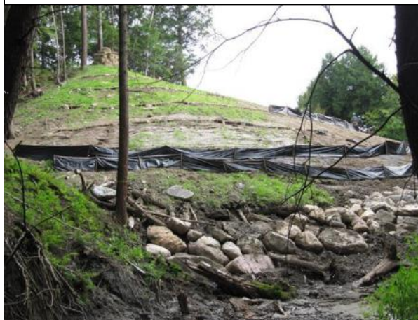
Figure 18. Before and two weeks after implementation: a bioengineering fix to a seriously eroding brook in Williston is taking hold. VYCC conducted the work.
